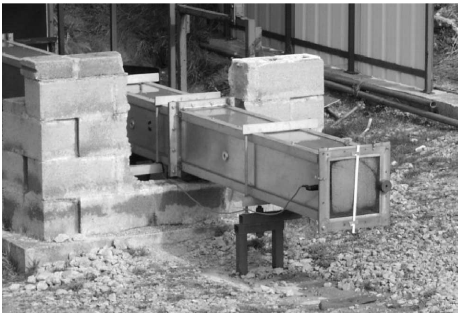
Fig. 11. Close-up of explosion duct showing vent cover that falls to ground immediately before ignition.
